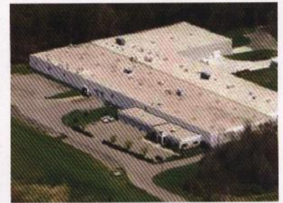
Tri-State Fabricators operates from this 125,000 square-foot facility near Cincinnati.
